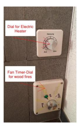
This burner is both wood-fired and electric.
